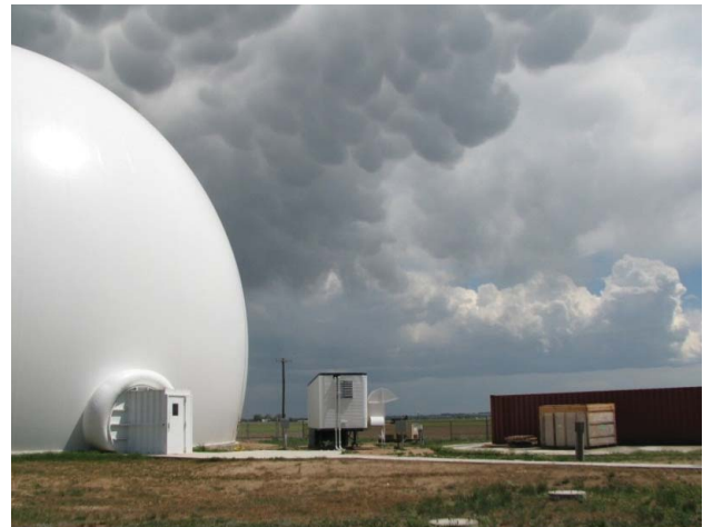
(Figure 2) The picture of the CSU-CHILL radar which is an advanced dual-polarization dual-frequency radar. This picture shows the typical condition that an environmental radar operates in. The big white dome is made of electromagnetically "almost transparent" material so that the radar is protected from the harsh environment such as snow, sleet, hail and heavy rain
