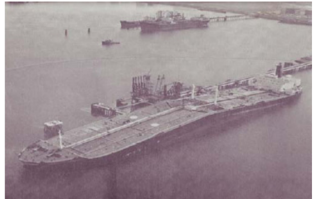
Fig. 3 Failure of EC
