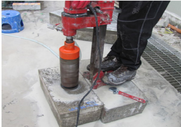
(a) Coring for Pull-Out Test
