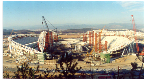
<Fig. 1> Bent method for keel truss
