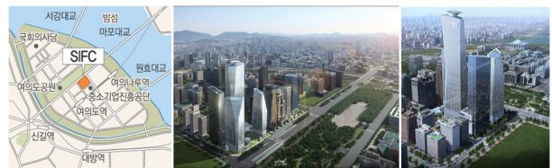
Fig. 2 Case building surroundings.
