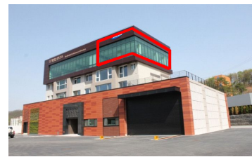
(a) Image of the building
