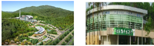
(a) Cheongju wide area incinerator (b) Purmi sports center
