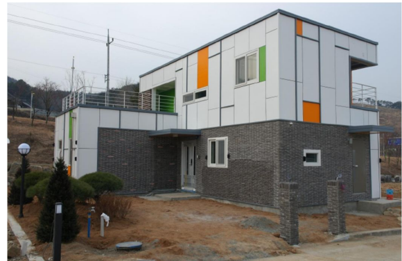
Fig. 1 Field Test House
