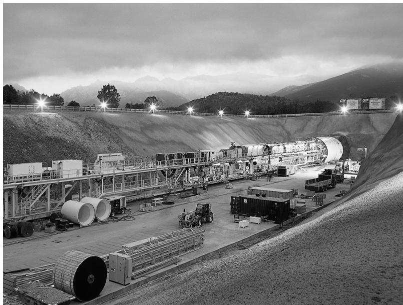
Fig. 5. The longest tunnel operated by High-power TBM in Guadarrama, Spain<sup>5)</sup>
