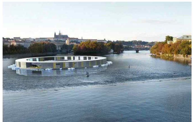
Fig. 5 Overview of floating pool
