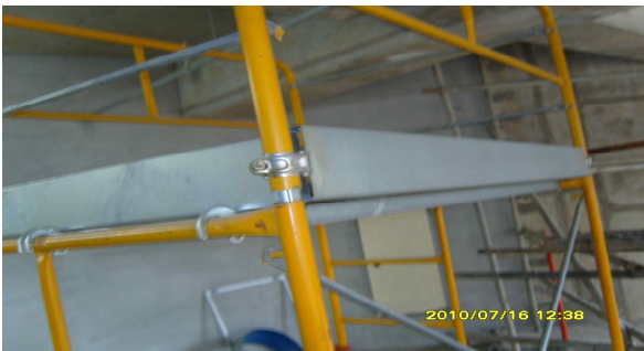
[Figure 2] Toe board of work platforms
