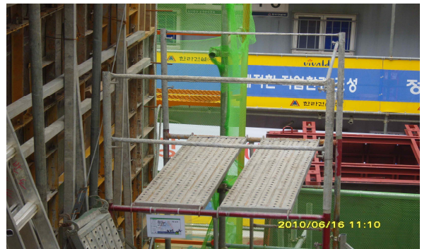
[Figure 1] Examples of work platforms of portable scaffold
