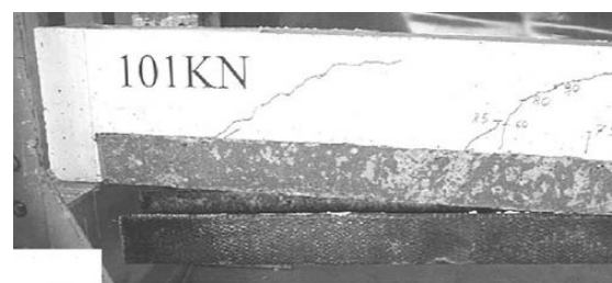
Fig. 5. Failure modes of Beam strengthened with wide width FRP (Brena et al, 2004)
