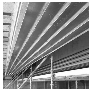
Fig. 1. Flexural strengthening of a reinforced concrete slab
