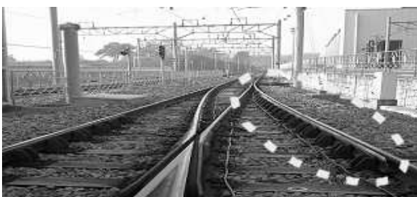
Fig. 3 Guard rails on Moonyang station – field survey
