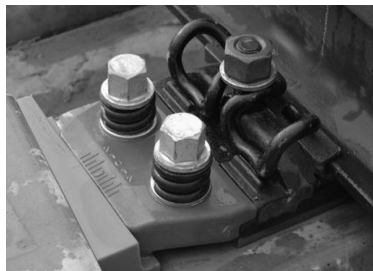
(a) SeoulMetro-Fastening system
