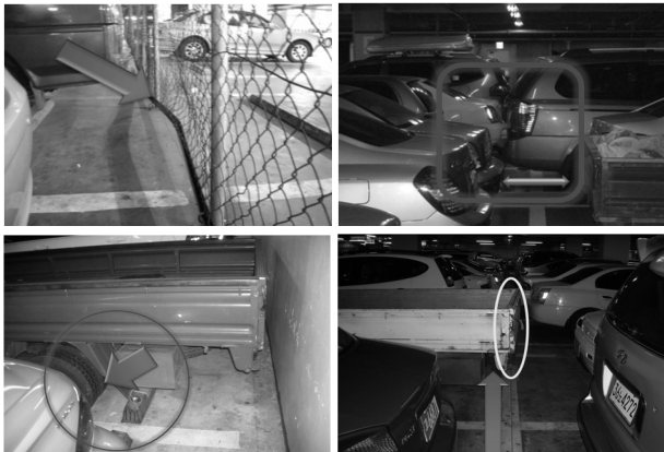
Fig. 6. Accident Cases Caused by Car-Stopper While Parked
