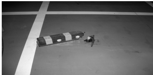
Fig. 9. Damaged Car-Stopper
