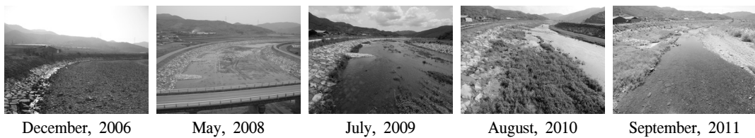
Figure 3. Field photographs of before and after spur dikes installation.
