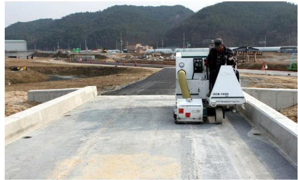
(a) Milling on the Surface of Bridge Deck
