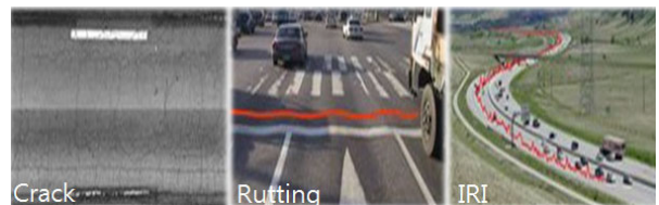
Fig. 1 The Influential Factors for the Determination of Pavement Condition Index (Crack, Rut Depth and IRI)
