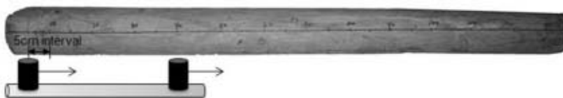
Fig. 5. Ultrasonic test method for replaced rafter member.
