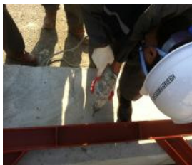
(a) Drilling of holes in concrete
