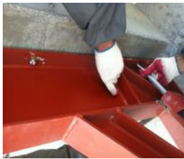
(c) Injection of sealant
