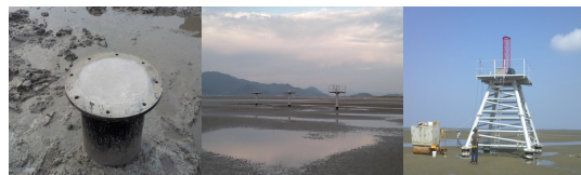
Fig. 7. Foundation & Substructure for Tower Supporting.
