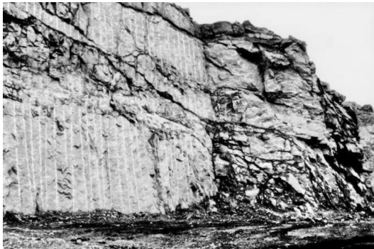
Fig. 7. Comparison between the results achieved by pre-splitting blasting (left) and normal blasting (right) for a surface excavation (Hoek & Brown, 1997).
