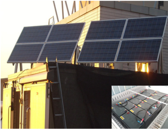
Fig. 3 Photovoltaic system for plant factory system.
