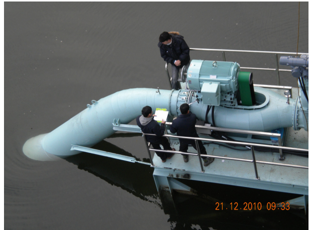
Fig. 5 Output Test of photos using by Penstock
