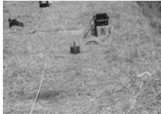
Fig. 3. Installation of accelerometer on the crest of the dam
