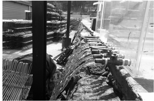
Fig. 7. Underground Runoff Measurement
