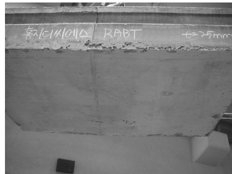
(a) Before Heating Test
