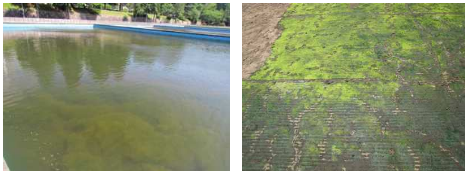
Fig. 1. Photographs of attached algae (left) and formed mat of algae (right) in the slow sand filters.
