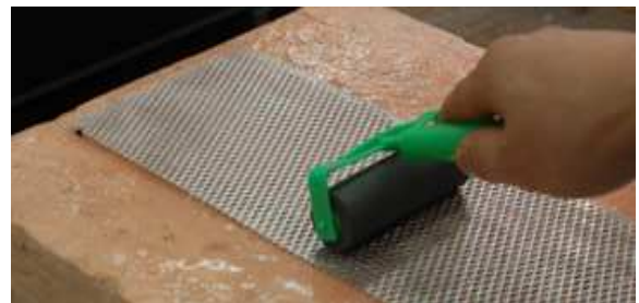
Fig. 2 Applying epoxy resin on the expanded metal core by using a roller
