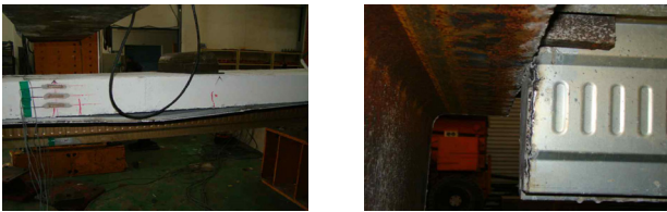
(a) Deck bonded failure (b) End slip
