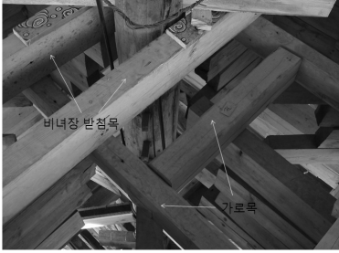
Fig.8 Floor Frame of Inside
