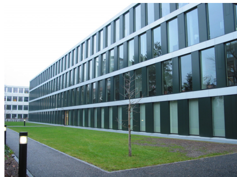
[Fig. 4] Bldg. of Winterthur Assurance, 2000, Burckhardt + Partner AG
