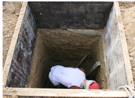
(b) Case 2 : A form is installed at the upper 0.4m foundation depth
