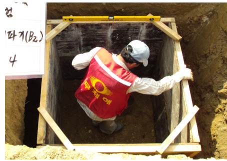
(a) Case 1 : A form is installed for the entire foundation depth
