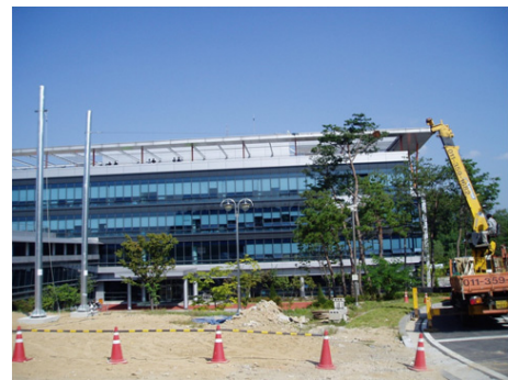
[Fig. 7] Loading method using a crane
