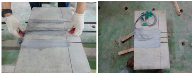
(c) Inserting of FRP plate (d) Finishing with epoxy mortar
