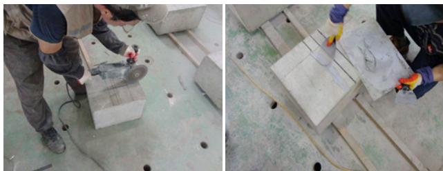
(a) Formation of grooves (b) Filling of epoxy mortar
