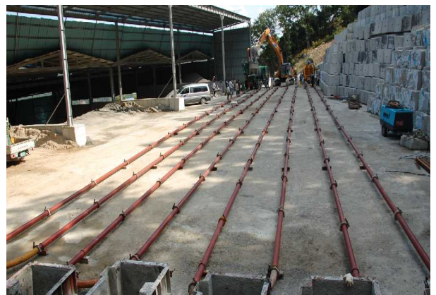
Figure 10. Horizontal pipe pumping test
