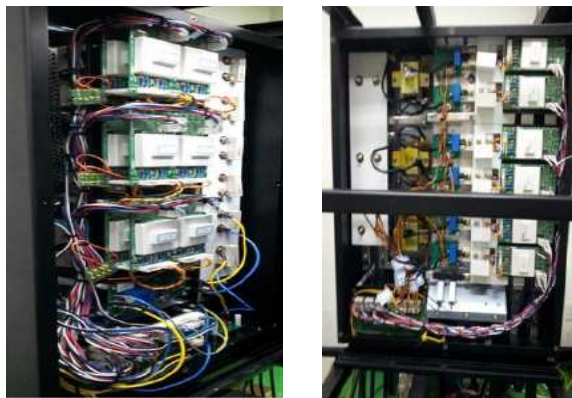
Fig. 13 Power stack built for the proto-type
