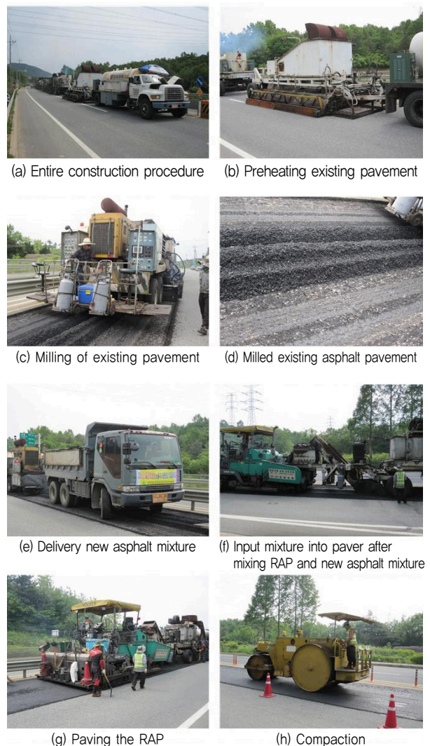
Fig. 1 HIR field construction
