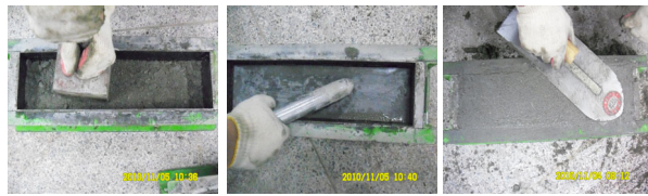
(a) Hammer drops 40times/layer (2 layers) (b) Vibration over steel plate 30sec/layer (2 layers) (c) Surface finish
