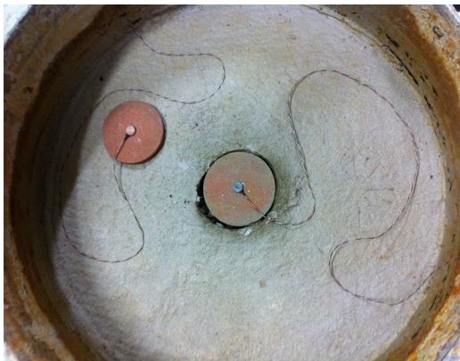
Fig. 8. Installation of earth pressure cell
