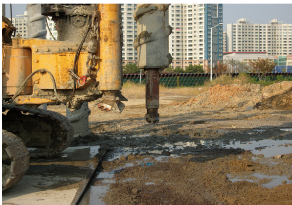
(b) Inner rod bit and pile bottom bit
