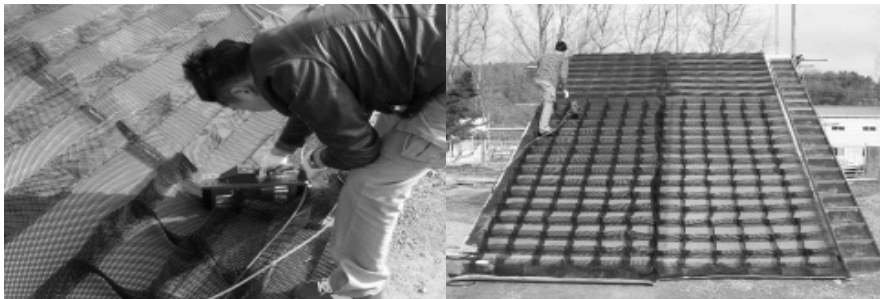
Fig. 3. GMC installation using the ultrasonic wave device
