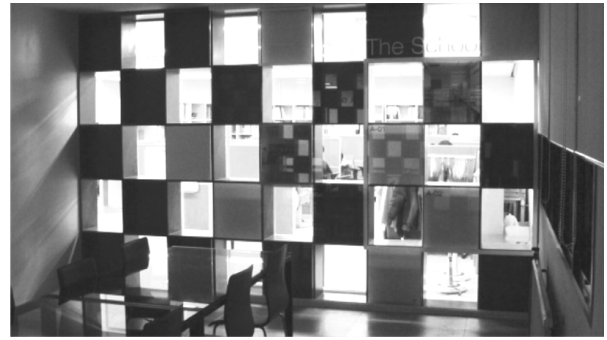
Fig. 4 Steel Grid Shear Wall
