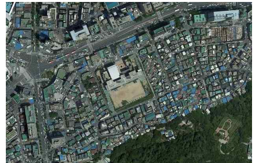
Fig. 6. Chang-cheon elementary & satellite picture
