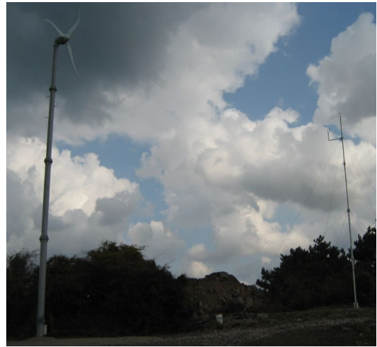
Fig. 1 Installed Skystream 3.7 with 10m high met mast
