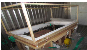
(a) Form work preparation
