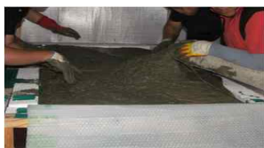
(c) Concrete pouring
