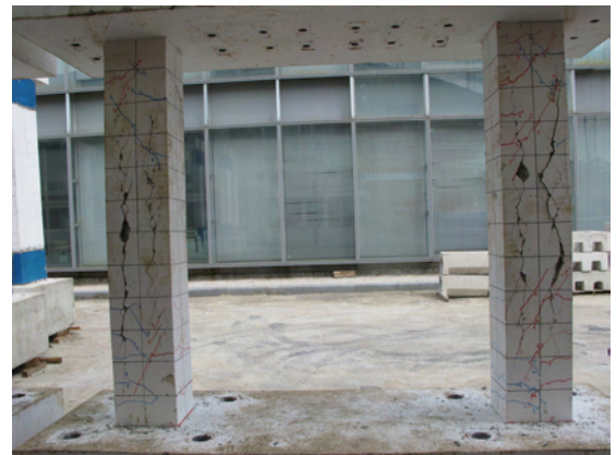
Fig. 5 Cracks that appeared following different loading steps for the CS-0 specimen
