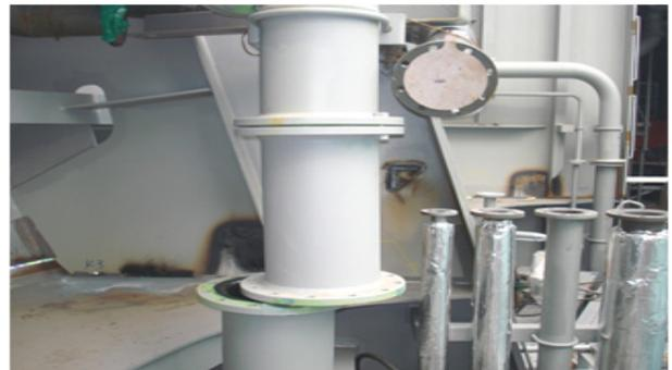
Fig. 1 Example of pipe support mismatch
