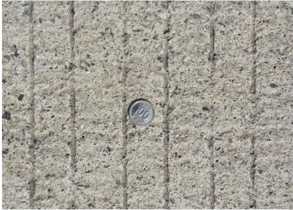
Fig. 5 Surface of Longitudinal Tining
