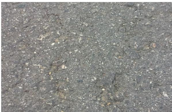
Fig. 7 Surface of Micro Surfacing
