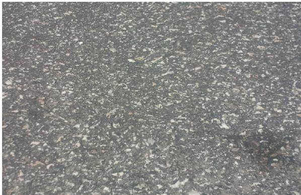
Fig. 6 Surface of Slurry Seal
