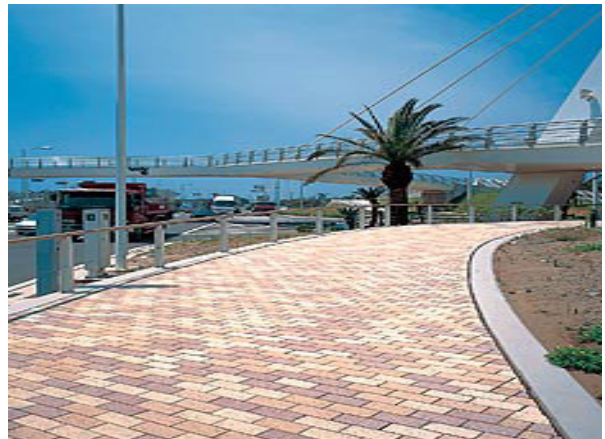
Fig. 5 Block Pavement for Japan Photocatalytic Concrete (Anne Beeldens et. al., 2006).
