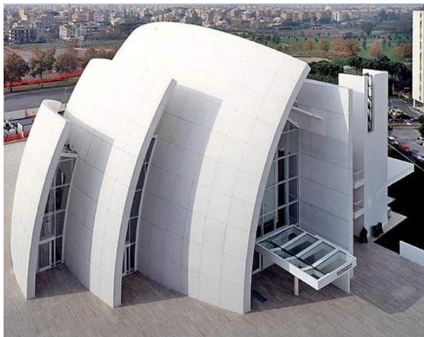
Fig. 4 TiO 2 -based Photocatalytic Cement for External to the Concrete of the City of Rome Jubilee Church Practices (Italcementi Group, 2007).
